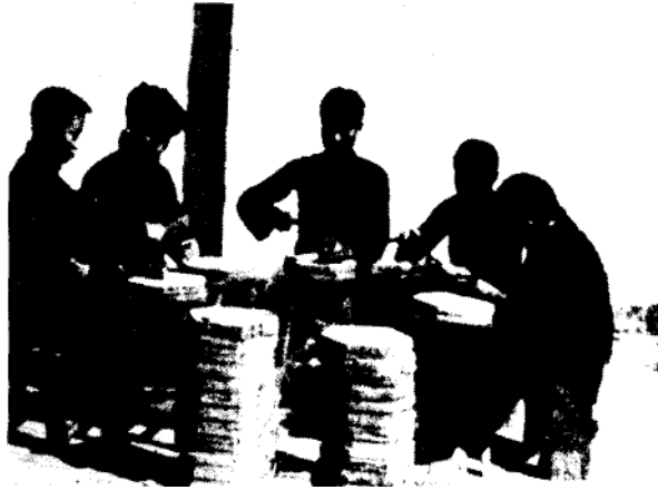
FIGURE 38. Crimping the Buck Ends of the Tubes. (Courtesy Wallace Clark.)
