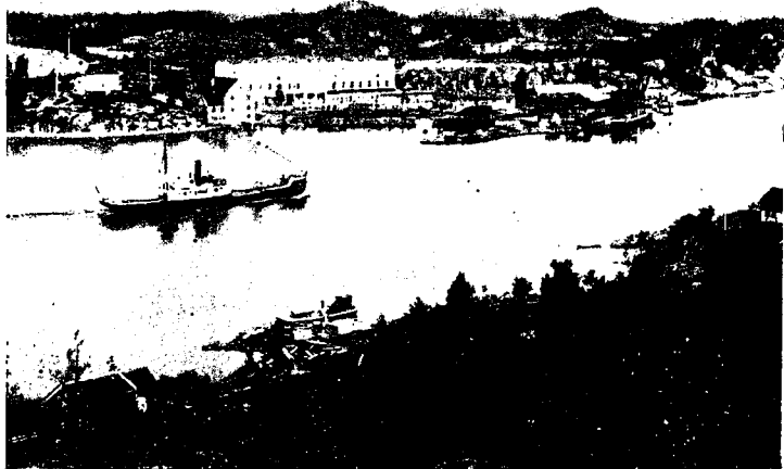
PHOTOGRAPH 1.—NORWEGIAN NITRIDES AND ALUMINIUM COMPANY. Works at Eydehavn near Arendal (25,000 H.P.), situated on an arm of the sea.
